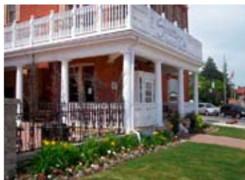
Railroad YMCA Building (c 1907)
